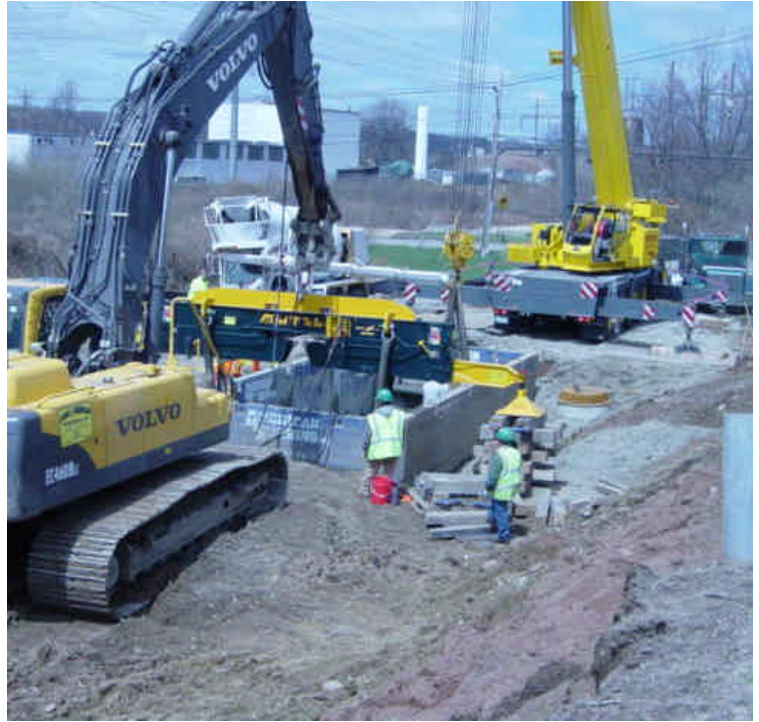
Photo of vault #5 construction activities.
