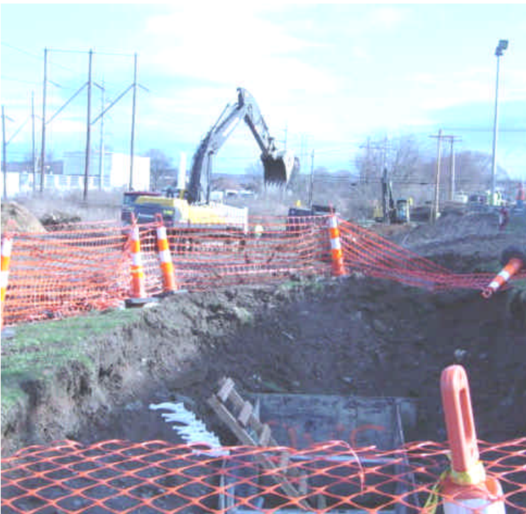
Photo of excavation activities for vault #5. Crews were actively removing and transporting environmentally sensitive soil to an adjacent, exposed slope should be temporarily or permanently approved location.
