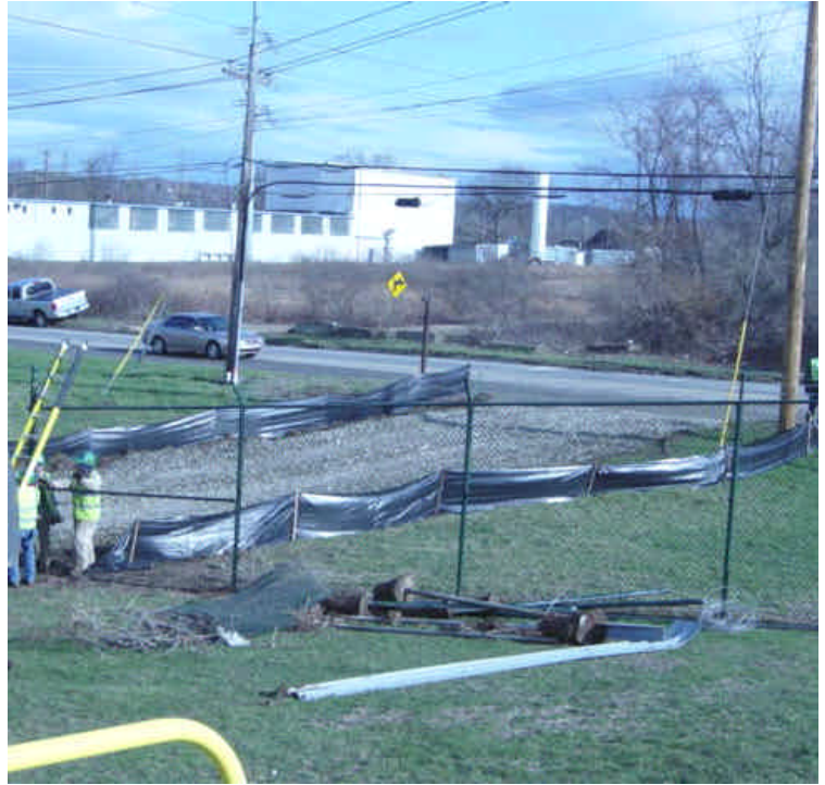
Photo of the construction entrance located at sta. #1080.
