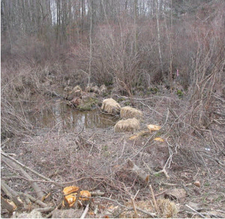
Area of the ROW that has been cleared south of Beseck SS off High Hill Rd. Low growing vegetation was retained in the wetlands here appropriately. Haybales left in wetlands for access should be removed.
