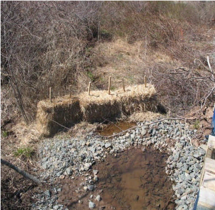
Stormwater controls installed adjacent to the timber mat crossing off Rte 17. Clear water was flowing off site.
