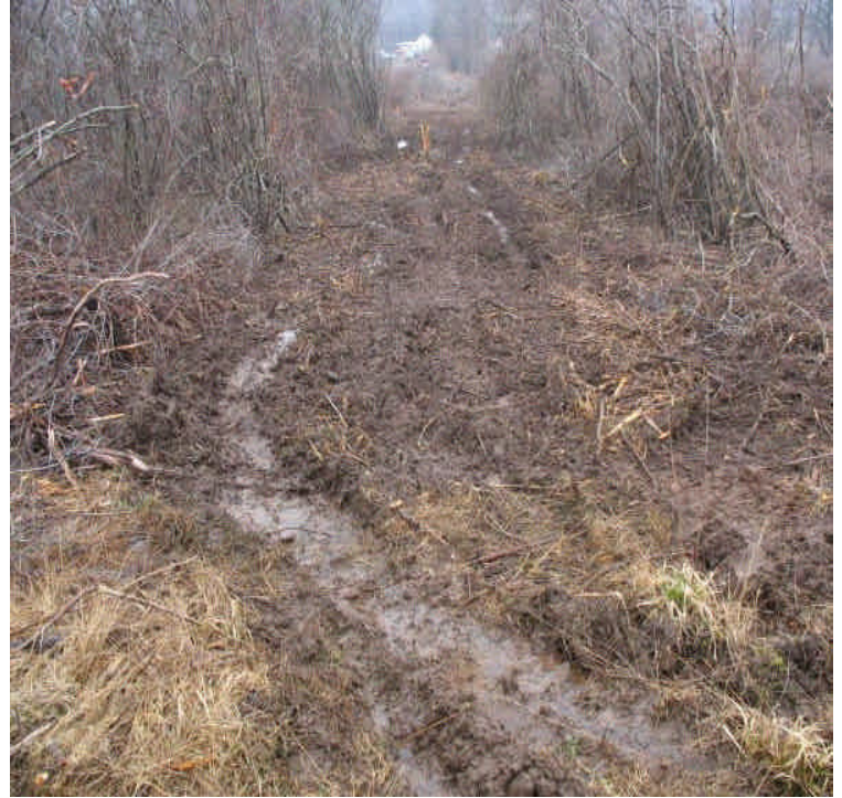
Ruts were observed from equipment through wetlands near Rte 17. Mats should be installed to support vehicles before they access saturated/wetland areas.
