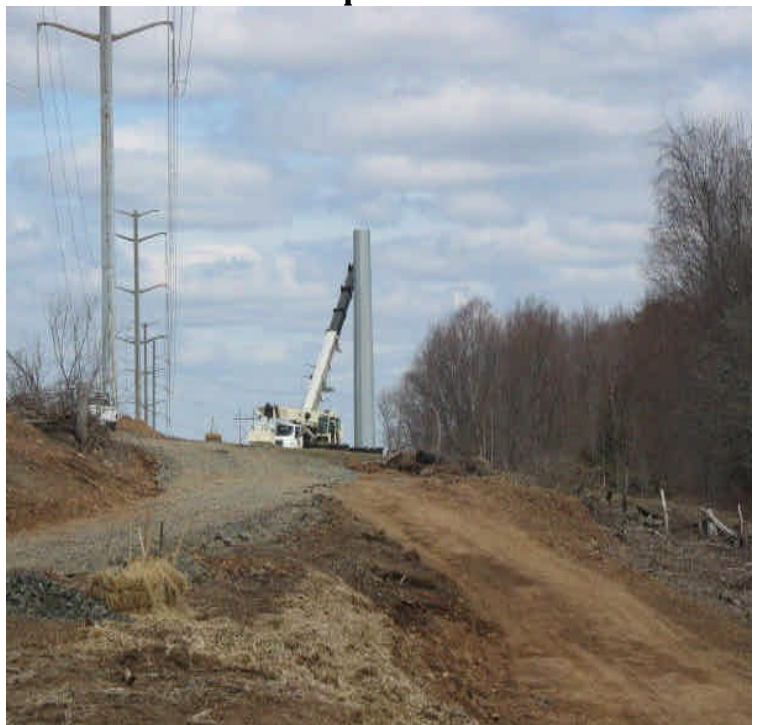
New pole construction was occurring just north of the Beseck SS.
