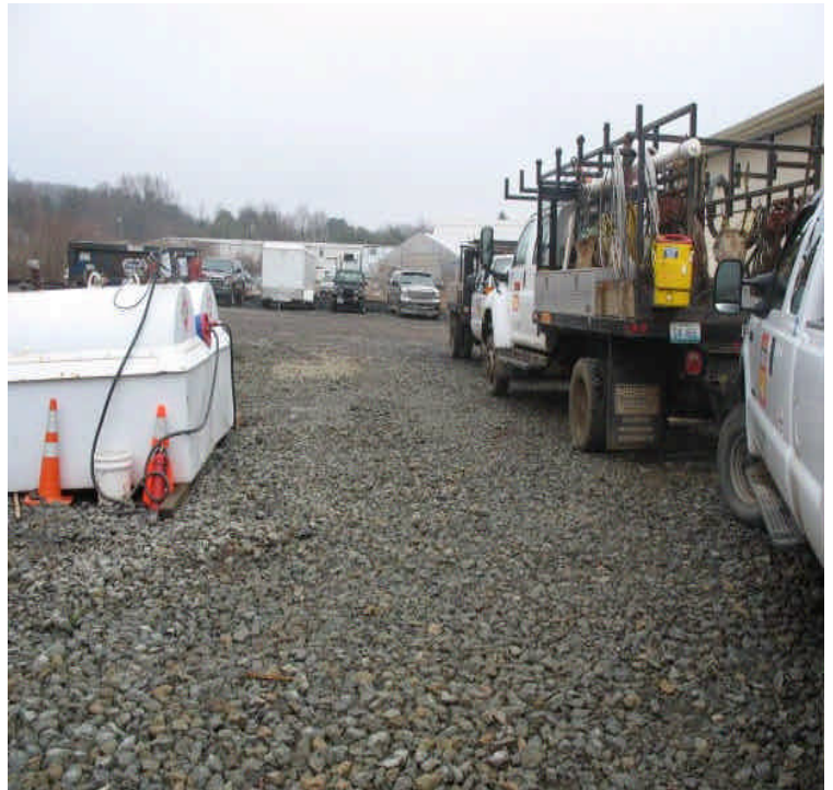
Both nozzles were contained at the fuel tanks within the contractor receiving yard. No spills were noted during this inspection.
