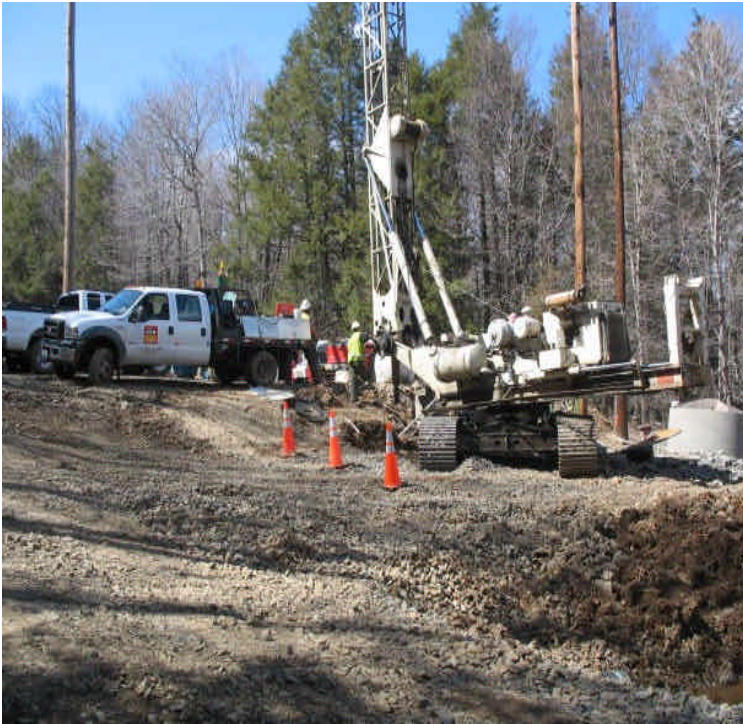
Foundations were being drilled off Powder Hill Rd.
