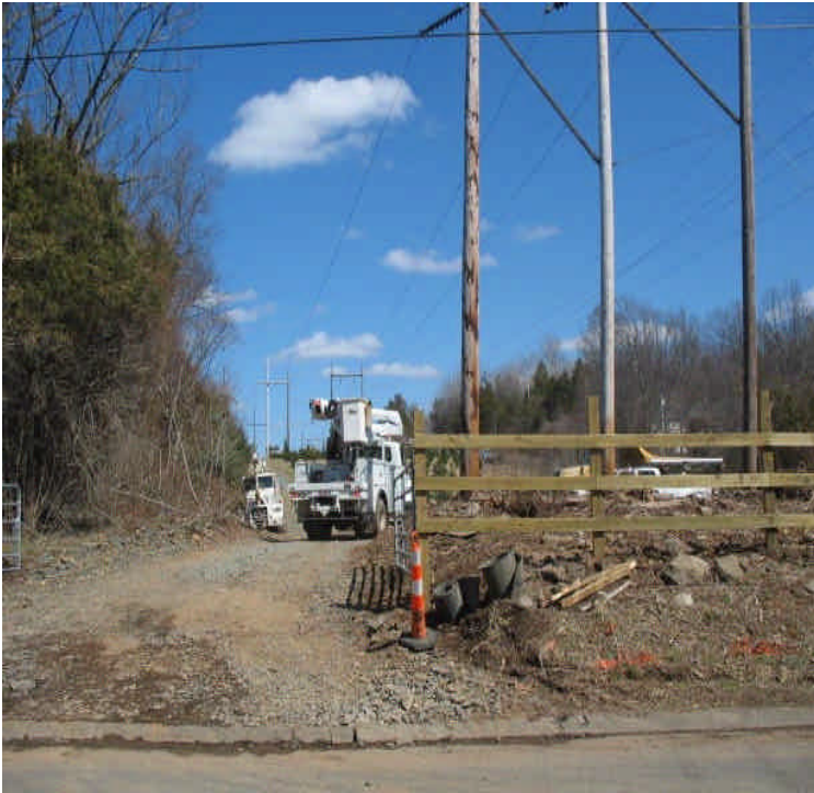
Line removal underway off Powder Hill Road.
