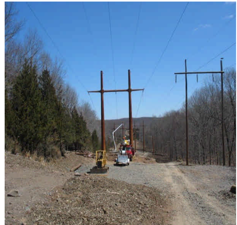
Line removal/installation continue off Black Walnut Dr.
