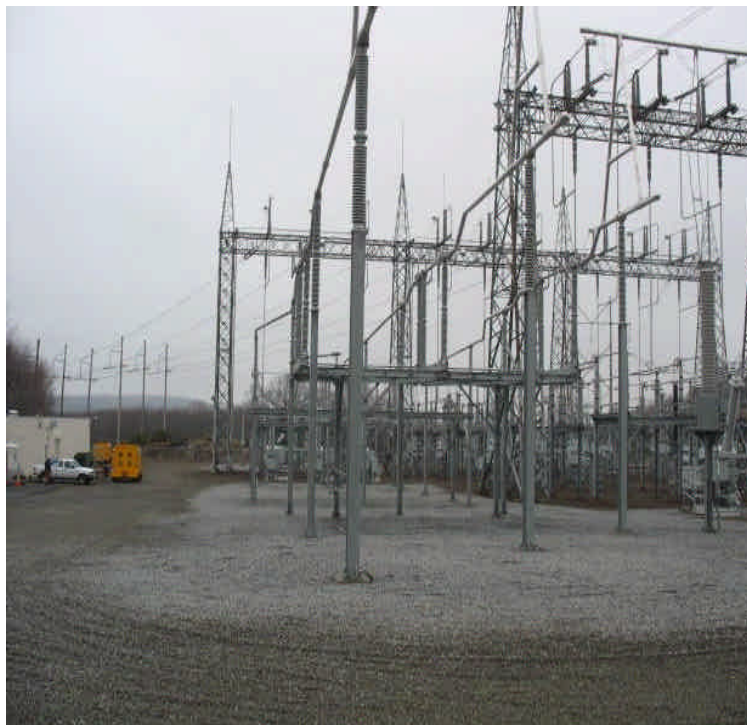
The site is stable and civil and structural work in the yard appears to be complete.
