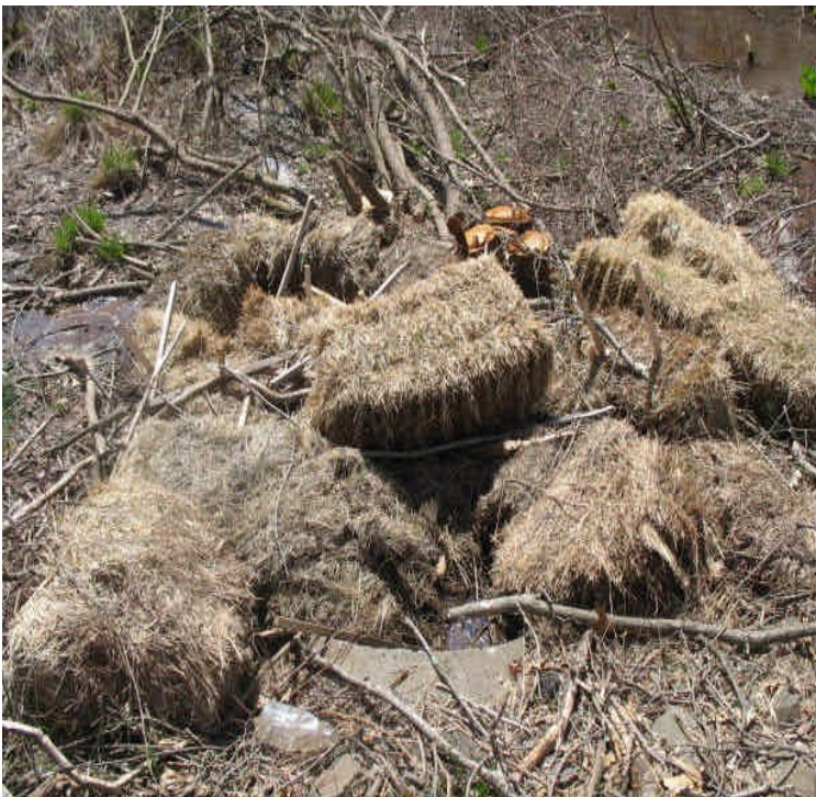
Storm drain outlet across Carpenter Lane has clear water flowing through the haybales.
