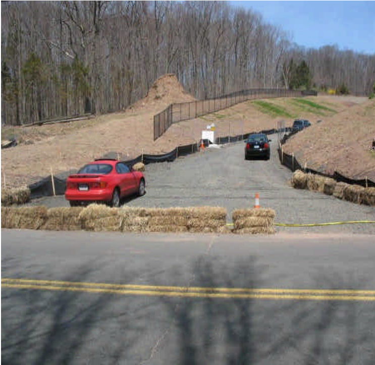
Site entrance off Carpenter Lane is well controlled; the area is being used for temporary parking of personal vehicles.
