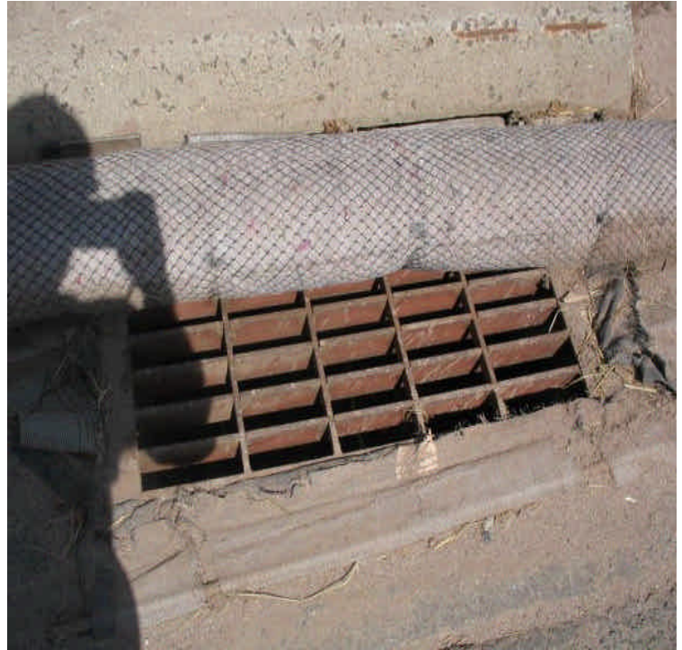
Carpenter Lane was recently swept and gutter buddies were cleaned and replaced in the catch basin.
