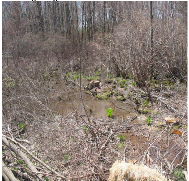
Clear water was observed leaving the haybales and entering the wetlands. Evaluate whether the amount of sediment accumulation justifies the minor disturbance needed to remove it, once the water subsides.
