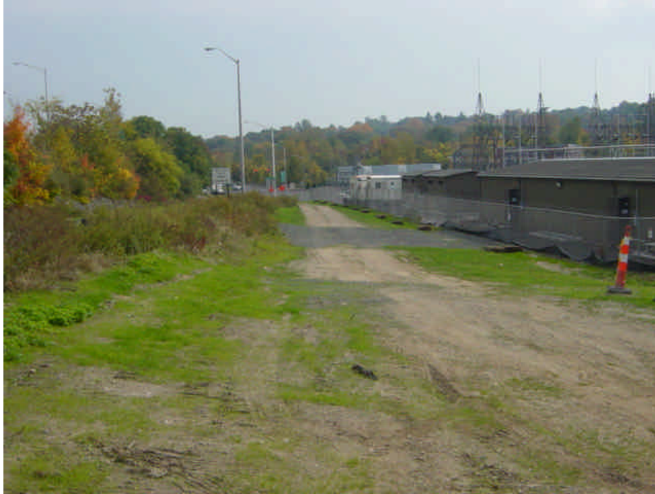
The area adjacent to the Norwalk substation near sta. #4-8 has been seeded and the area is beginning to vegetate, except in some areas where construction traffic is impeding vegetation growth. The drainage swale has been restored, but sediment has washed out and accumulated in portions of the swale.
