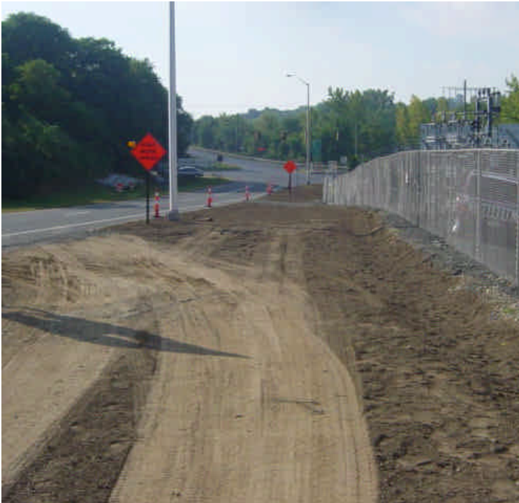
Area between sta #2-9 has been re-graded to restore the drainage swale along the side of the substation. Exposed topsoil will need to be stabilized. The area around the drainage inlet at sta. #9+50 has also been re-graded. Temporary controls are needed until the area stabilizes.
