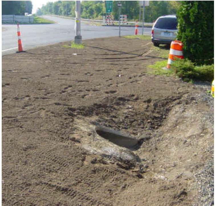
Area between sta #2-9 has been re-graded to restore the drainage swale along the side of the substation. Exposed topsoil will need to be stabilized. The area around the drainage inlet at sta. #9+50 has also been re-graded. Temporary controls are needed until the area stabilizes.
