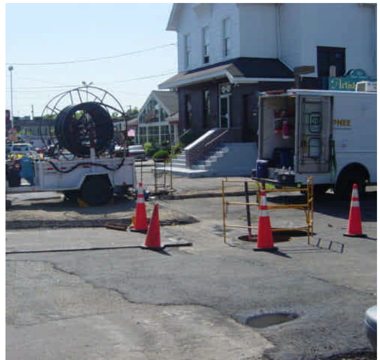
Trenching continues in various locations between sta. #31-34 & #38. Steel plates were covering the trench at the time of the inspection. A minor amount of cold mix/ granular material was observed along the edge of the roadway. Electrical contractor was on site at vault # 3.
