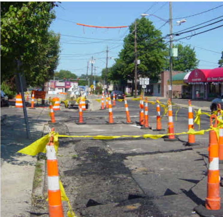
Trenching continues in various locations between sta. #31-34 & #38. Steel plates were covering the trench at the time of the inspection. A minor amount of cold mix/ granular material was observed along the edge of the roadway. Electrical contractor was on site at vault # 3.
