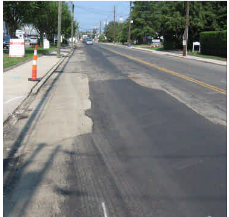
Trenching continues in various locations between sta. #31-34 & #38. Steel plates were covering the trench at the time of the inspection. A minor amount of cold mix/ granular material was observed along the edge of the roadway. Cold mix/ granular material along the roadway between sta. #38-45 appears to have been swept.
