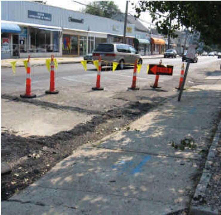
Trenching continues in various locations between sta. #31-34 & #38. Steel plates were covering the trench at the time of the inspection. A minor amount of cold mix/ granular material was observed along the edge of the roadway. Cold mix/ granular material along the roadway between sta. #38-45 appears to have been swept.
