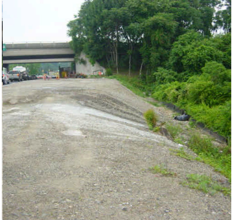
Sediment and debris continues to accumulate along the silt fence near sta. #14-16. Gullies have formed in several areas and portions of the slope are beginning to erode. Evidence of multiple concrete washouts were also observed since 6/27. There is no active work in this area and it is unclear whether the washouts are project related. This area needs to be restored/stabilized per the D&M timelines.
