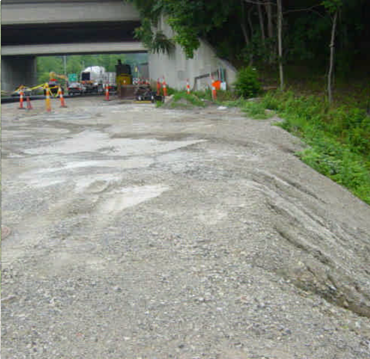
Sediment and debris continues to accumulate along the silt fence near sta. #14-16. Gullies have formed in several areas and portions of the slope are beginning to erode. Evidence of multiple concrete washouts were also observed since 6/27. There is no active work in this area and it is unclear whether the washouts are project related. This area needs to be restored/stabilized per the D&M timelines.
