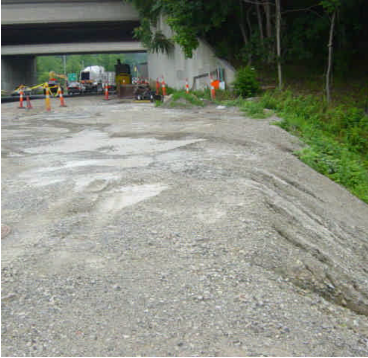
Sediment and debris continues to accumulate along the silt fence near sta. #14-16. Gullies have formed in several areas and portions of the slope are beginning to erode. Evidence of multiple concrete washouts were also observed. There is no active work in this area and it is unclear whether the washouts are project related. This area needs to be restored/stabilized per the D&M timelines.
