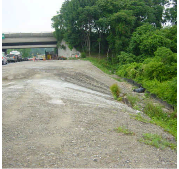
Sediment and debris continues to accumulate along the silt fence near sta. #14-16. Gullies have formed in several areas and portions of the slope are beginning to erode. Evidence of multiple concrete washouts were also observed. There is no active work in this area and it is unclear whether the washouts are project related. This area needs to be restored/stabilized per the D&M timelines.
