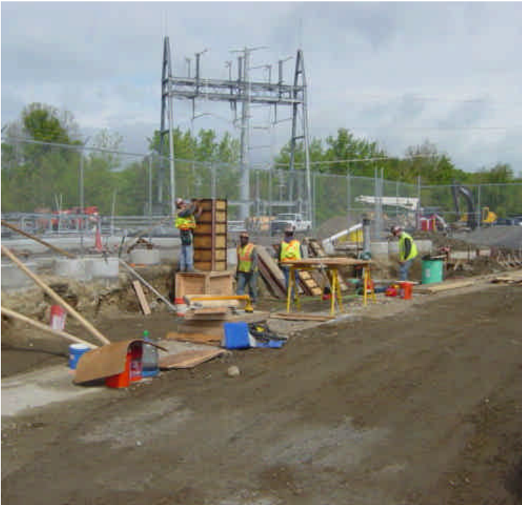
Crews were forming foundations around the conduits to terminate each of the circuits at the Norwalk substation.
