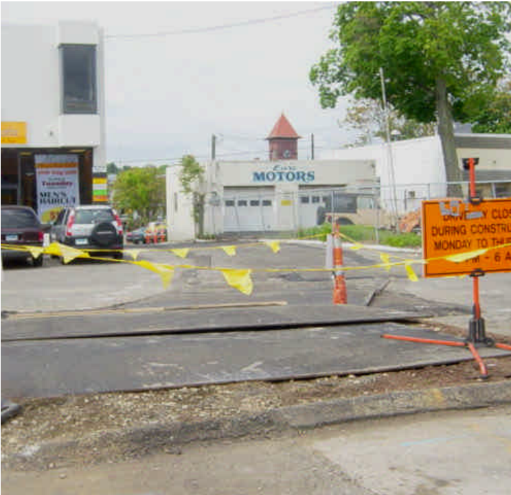
Steel plates remain in place over the trench near sta. #28-30.
