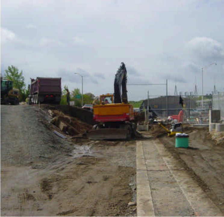
Backfilling work was ongoing near sta. #0-2. The pre-cast concrete retaining wall was temporarily removed to facilitate trenching work.
