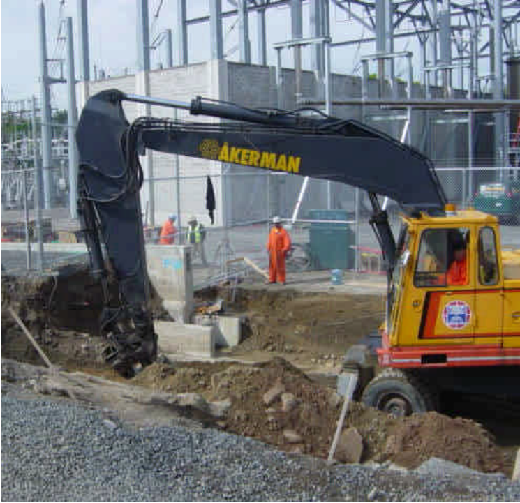
Backfilling work was ongoing near sta. #0-2. The pre-cast concrete retaining wall was temporarily removed to facilitate trenching work.
