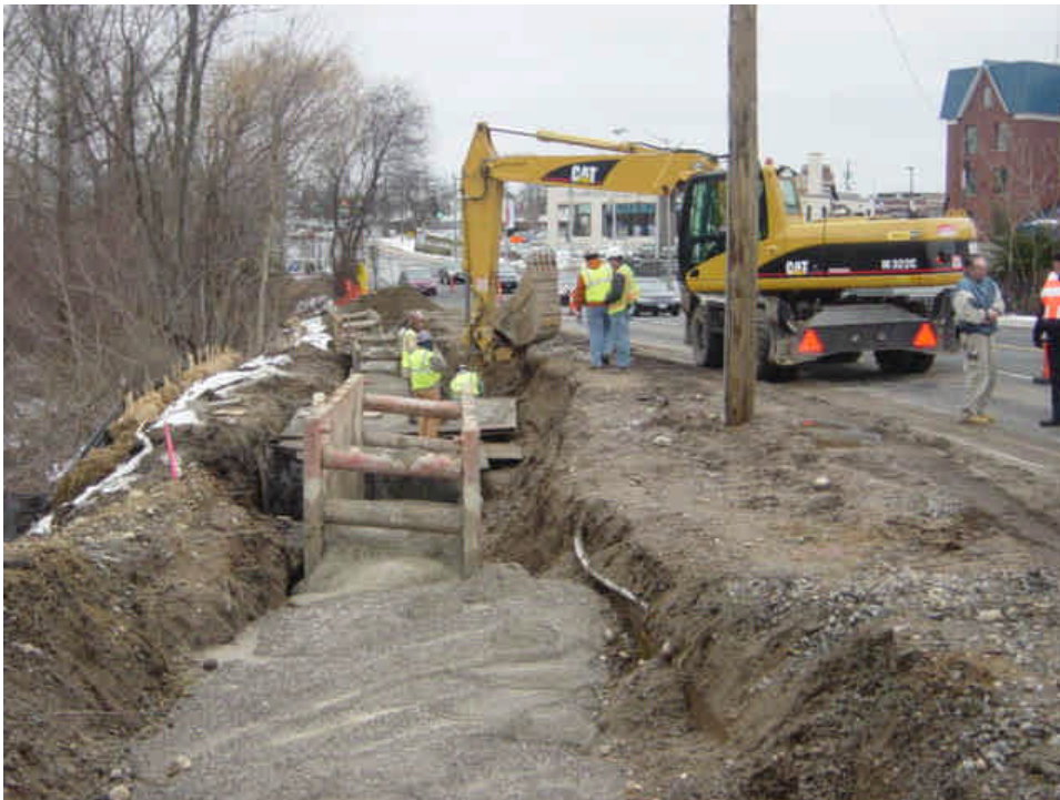
At stations #16-17, trenching and backfilling continue.
