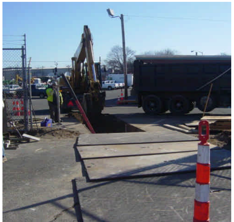
Trenching activities continue near sta. #24-25.
