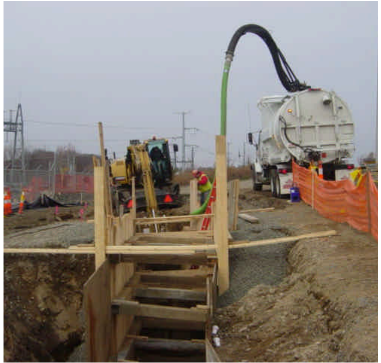
Trenchwork continues near sta. #4 along the substation fence and Rt. 7 off-ramp.
