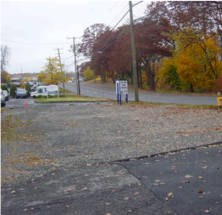
The area near vault #11 has been partially restored.
