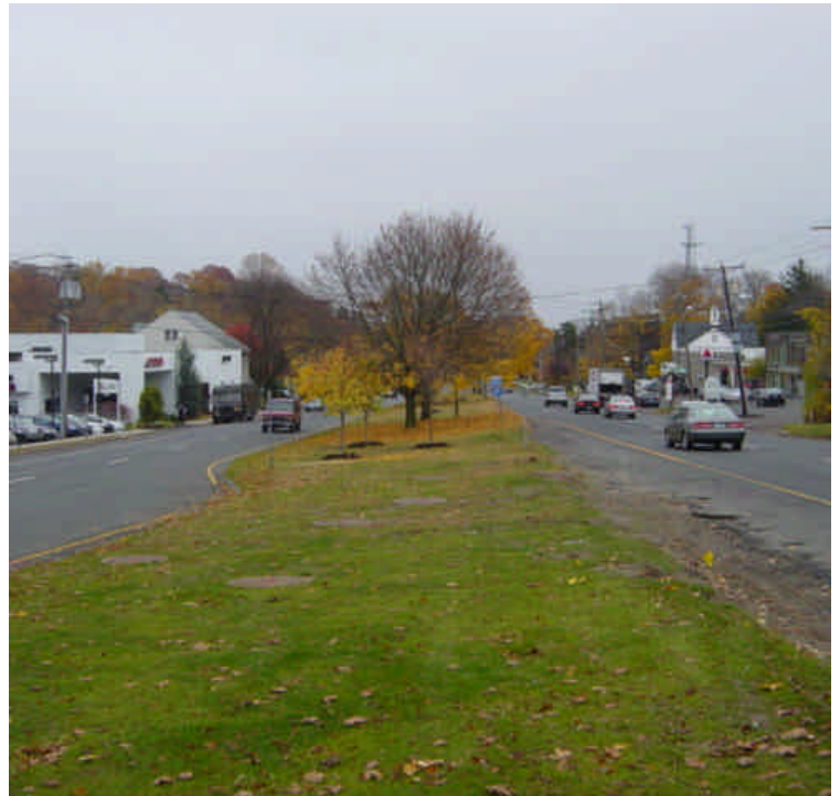
The area near sta. #316-318 has been partially restored. Trees have been planted in the median area. Some ruts remain in a few locations and bituminous curbing still needs to be restored. Damage along the edge of the roadway also needs repair.
