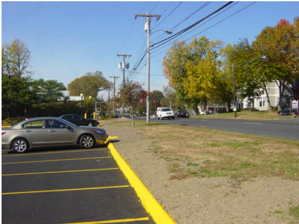
Area near vault #26 has been restored and portions of the area are beginning to revegetate. Ensure areas of exposed soil are stable prior to the winter.
