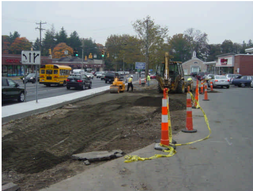
Restoration efforts were underway near sta. #283-284 at vault #17.
