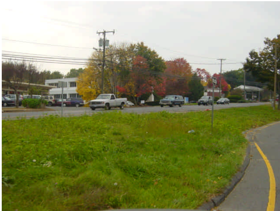
The area near sta. #316-318 has vegetated with weedy growth and grass cover. Bituminous curbing still needs to be restored in this area.
