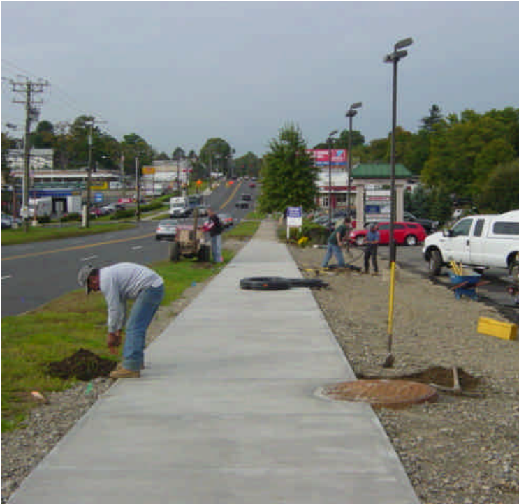
Restoration work was underway near sta. #129-131 and vault # 8.
