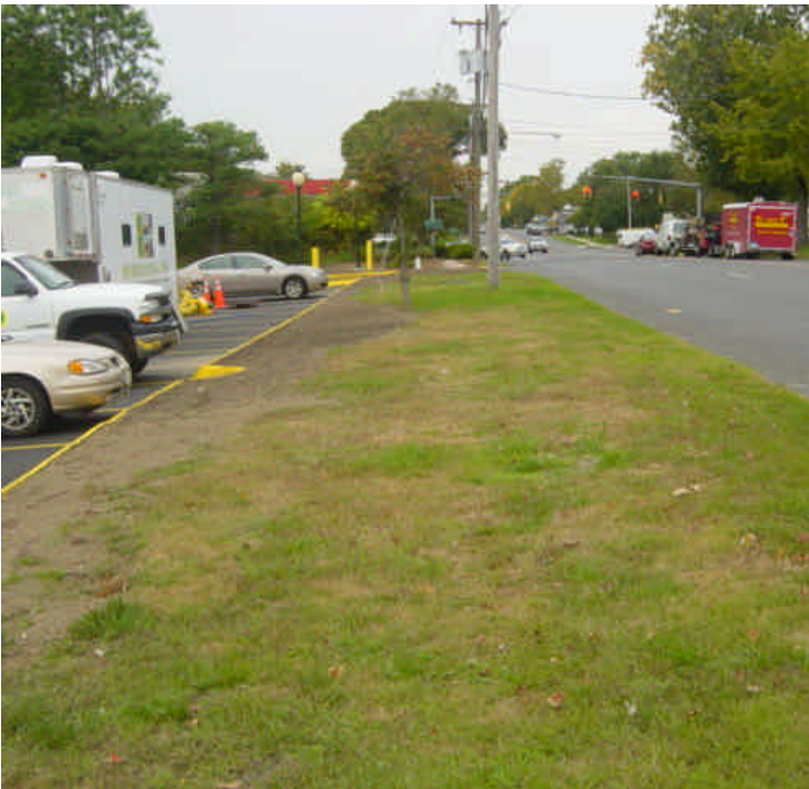
New River Electric was on site at vault #26.
