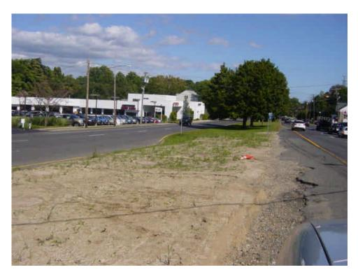
Topsoil has been spread in the area near sta. #316-318 but was not mulched. Minor gullies have formed in some locations due to heavy rains. Repair the erosion and apply mulch over the entire area.
