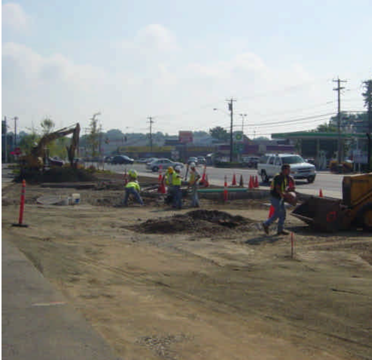
Restorations efforts were ongoing at sta. #146-148. Manhole rims were being adjusted and the area was being re-graded. Topsoil was spread in some areas. Provide mulch and seed to stabilize the soils.
