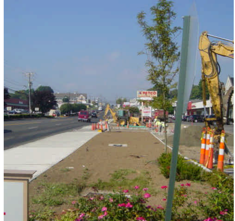
Restorations efforts were ongoing at sta. #146-148. Manhole rims were being adjusted and the area was being re-graded. Topsoil was spread in some areas. Provide mulch and seed to stabilize the soils.
