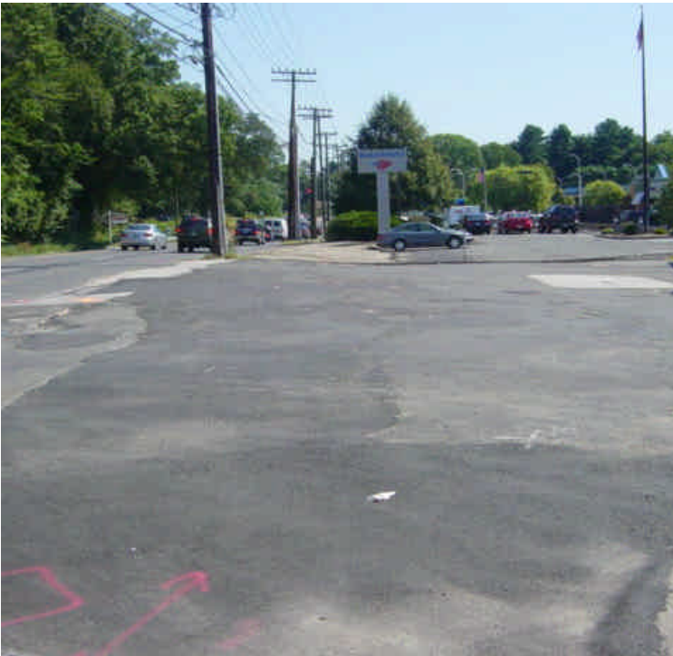
Tie-in work appears to have been completed at vault #10.
