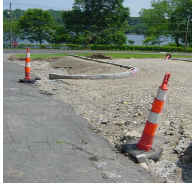
Stone curbing has been set near sta. #234. The adjacent areas have been partially re-graded and some of the material had eroded and accumulated at the intersection of Lincoln St. and Riverside Ave.
