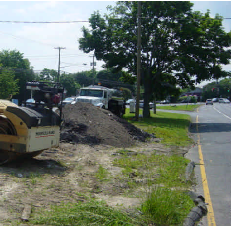
Sediment tracking and heavy rutting remains in the island near sta. #316-318. Paving contractor has begun parking equipment in this area. Active work has been complete for several months and restoration is needed. If material stockpiles are to be stored longer than one work day, controls should be installed.
