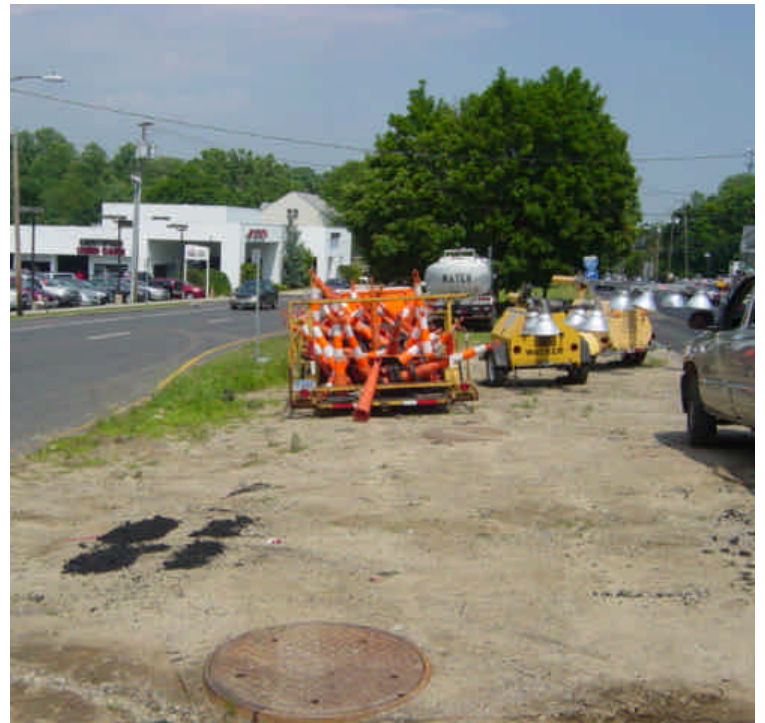
Sediment tracking and heavy rutting remains in the island near sta. #316-318. Paving contractor has begun parking equipment in this area. Active work has been complete for several months and restoration is needed. If material stockpiles are to be stored longer than one work day, controls should be installed.
