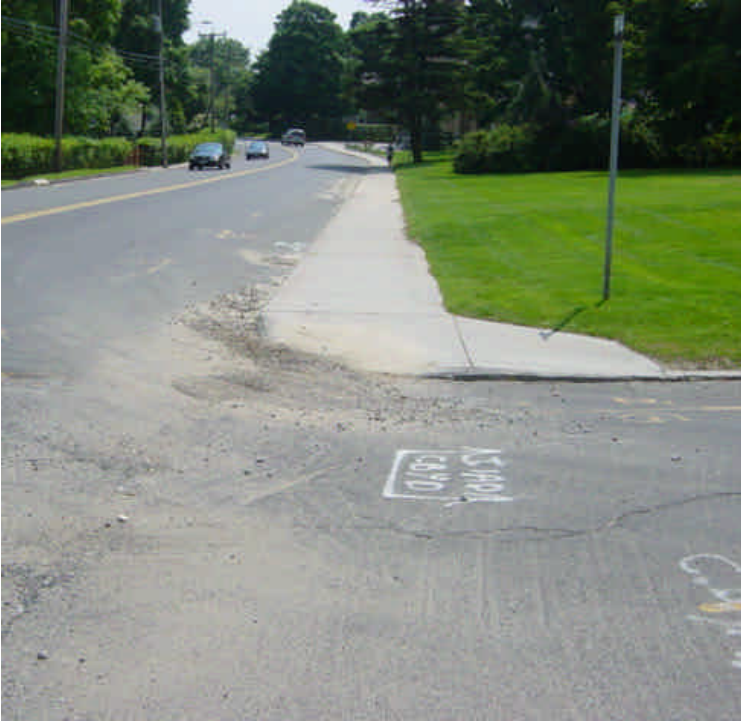
Stone curbing has been set near sta. #234. The adjacent areas have been partially re-graded and some of the material had eroded and accumulated at the intersection of Lincoln St. and Riverside Ave.
