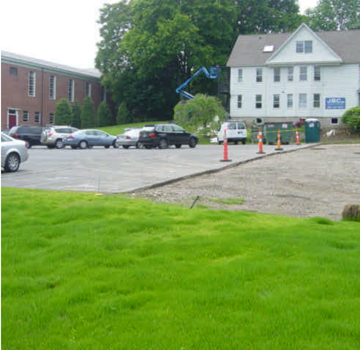
Vehicles are traveling through the exposed soil near sta. #234 and tracking sediment onto Lincoln St. as well as the adjacent parking lot area. This area has been scheduled for paving for some time.
