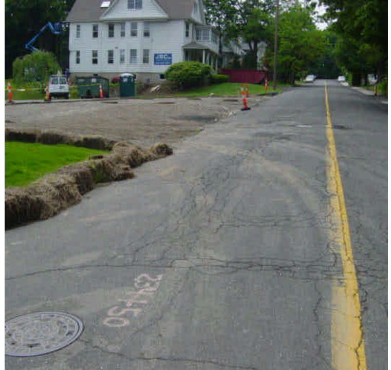
Vehicles are traveling through the exposed soil near sta. #234 and tracking sediment onto Lincoln St. as well as the adjacent parking lot area. This area has been scheduled for paving for some time.
