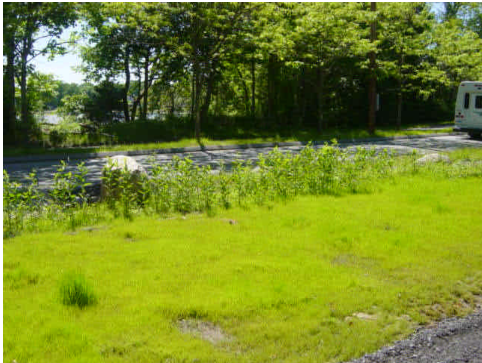
The area near sta. #252 was previously restored and a berm was constructed and vegetated along the entrance drive. The berm has been removed and additional gravel material spread in some areas. This work appears to have been completed by the town.
