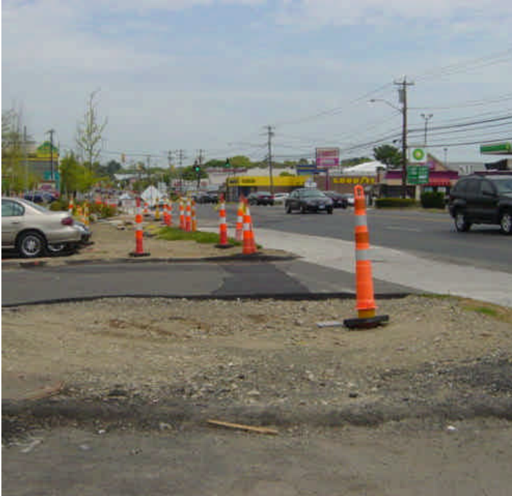
Trenching and vault tie-in work continues near sta. #148-149.
