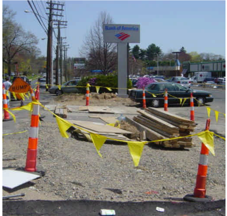
Vault tie-in work continues near sta. #163-166.
