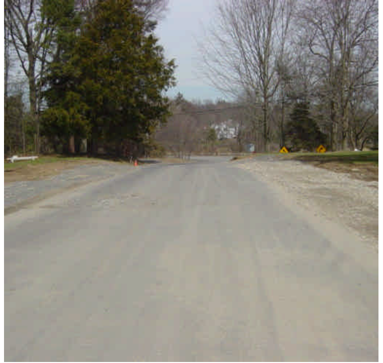
The access drive to the Sherwood Island yard appears to have been recently swept and sediment tracking was not observed this week.
