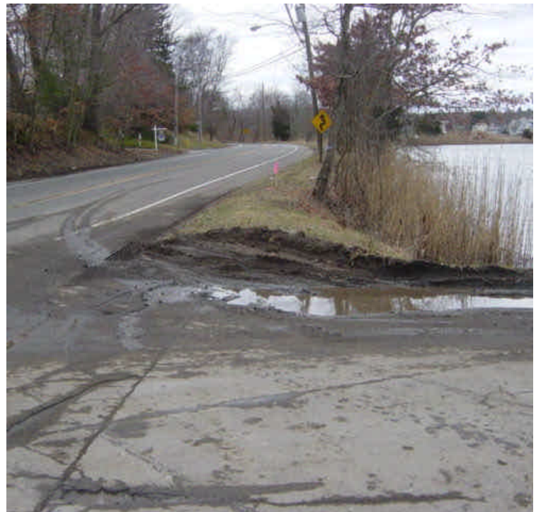
The construction entrance near the staging area on the east side of the Saugatuck River near sta. #251 is covered with mud and sediment and no longer functions. Sediment tracking was observed throughout the adjacent parking area. Heavy ruts have also formed near the corner of the access drive and Imperial Ave. The adjacent catch basin was not protected. Minor tracking was observed along Imperial Ave. but the area was being swept during the inspection. The entrance pad should be refreshed.
