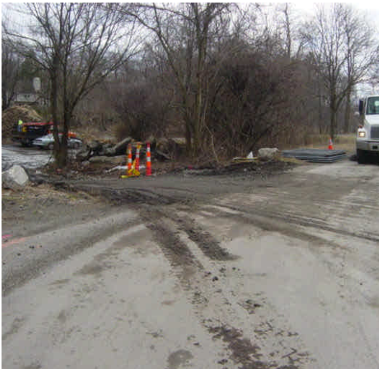
The construction entrance near the staging area on the east side of the Saugatuck River near sta. #251 is covered with mud and sediment and no longer functions. Sediment tracking was observed throughout the adjacent parking area. Heavy ruts have also formed near the corner of the access drive and Imperial Ave. The adjacent catch basin was not protected. Minor tracking was observed along Imperial Ave. but the area was being swept during the inspection. The entrance pad should be refreshed.
