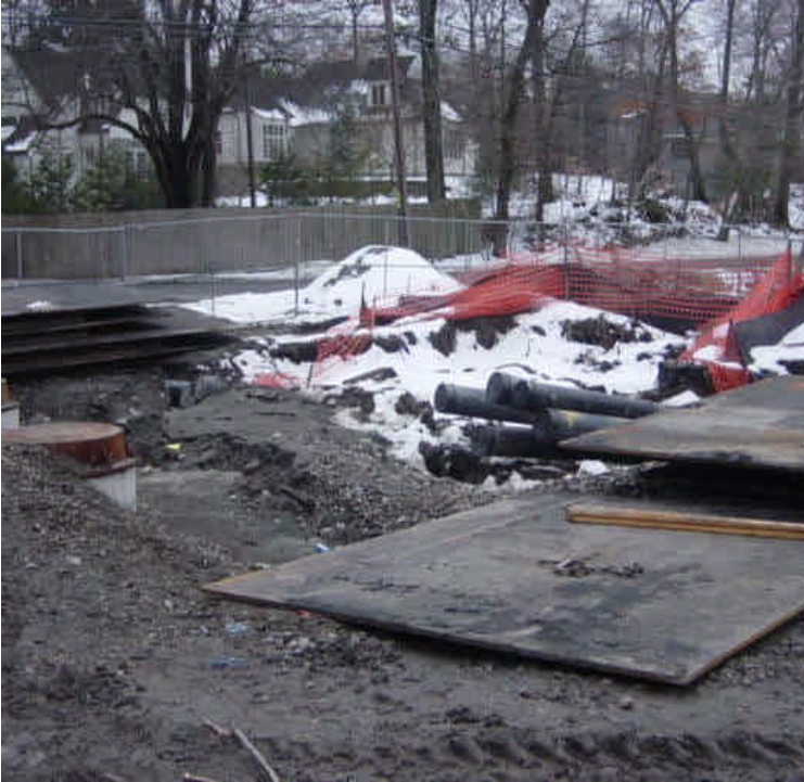
Vault #15 has been installed along Imperial Ave., near sta. #251.
