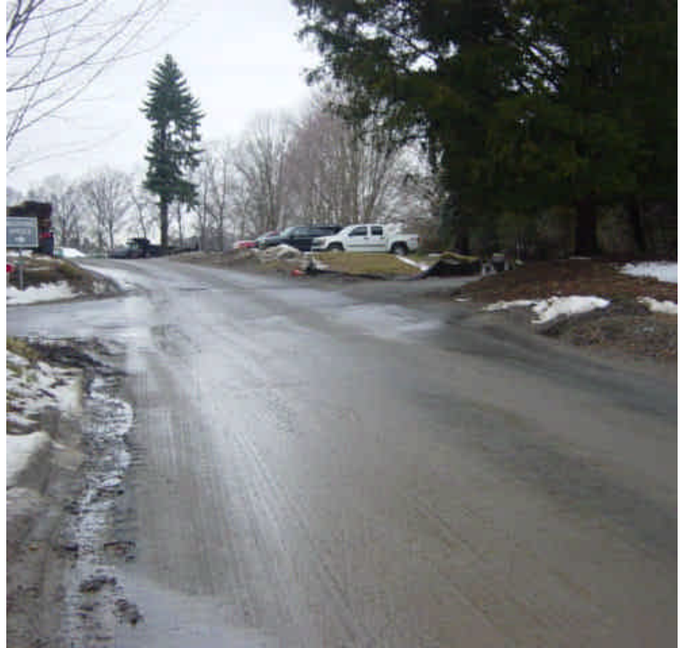
Sediment tracking continues to be noted along the access road to the Sherwood Island yard.
