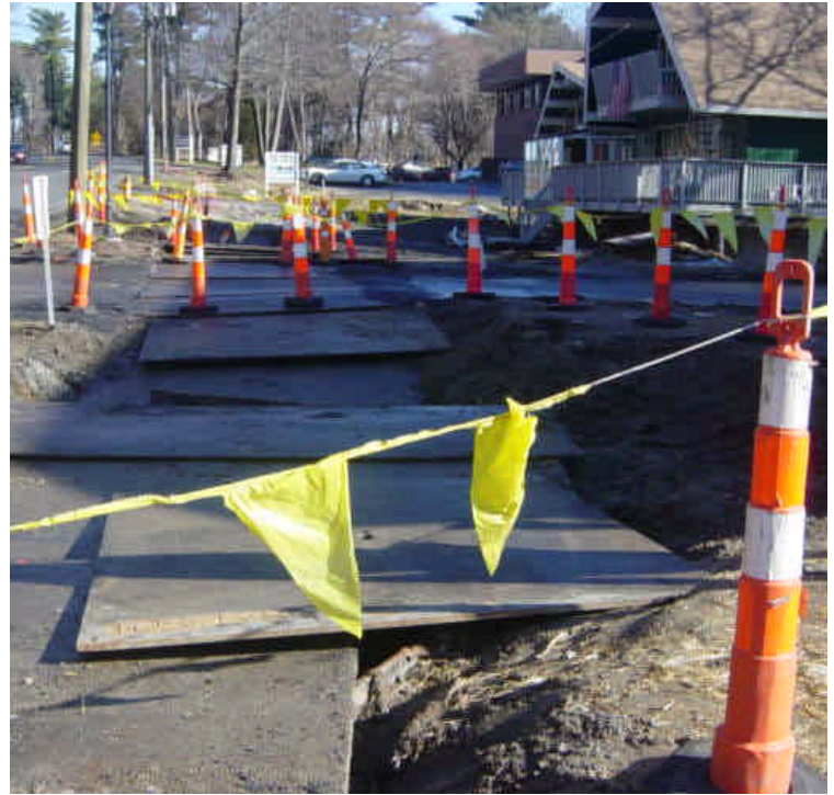
Steel plates are in use at the tie-in to vault 11 (stations #184-185).
