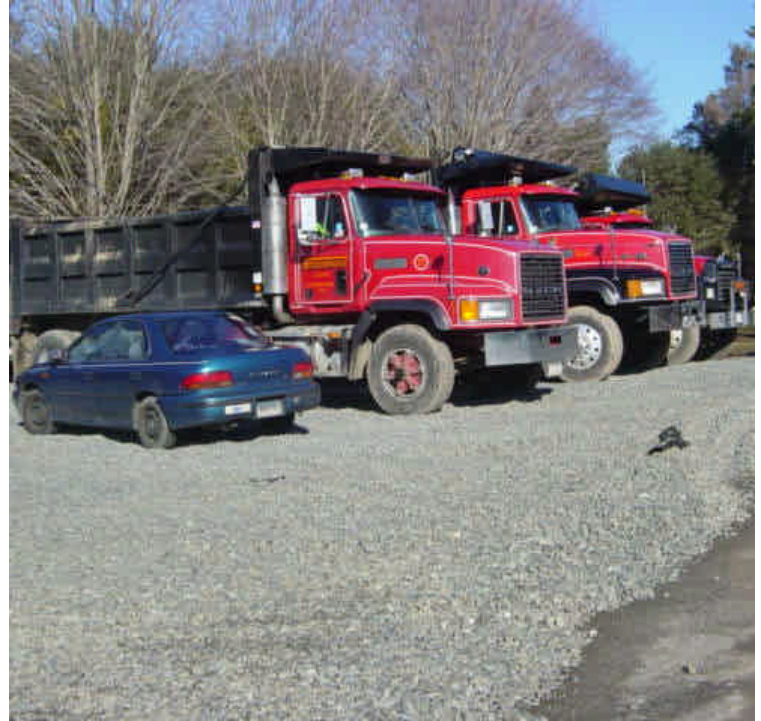
Along the sides of the Sherwood Island access road, more crushed stone has been installed in the area where heavy equipment has been stored, reducing ruts and tracking. Ensure that pre-construction conditions/surfaces are restored when the area is no longer in use.
