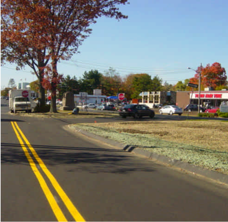
Topsoil has been spread near sta. #463 and the area has been hydroseeded. Bulbs were also being planted in the area.
