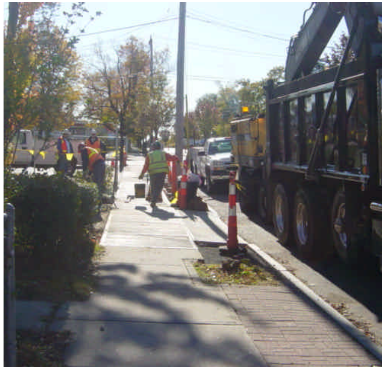
Sidewalk restoration was ongoing near sta. #695.
