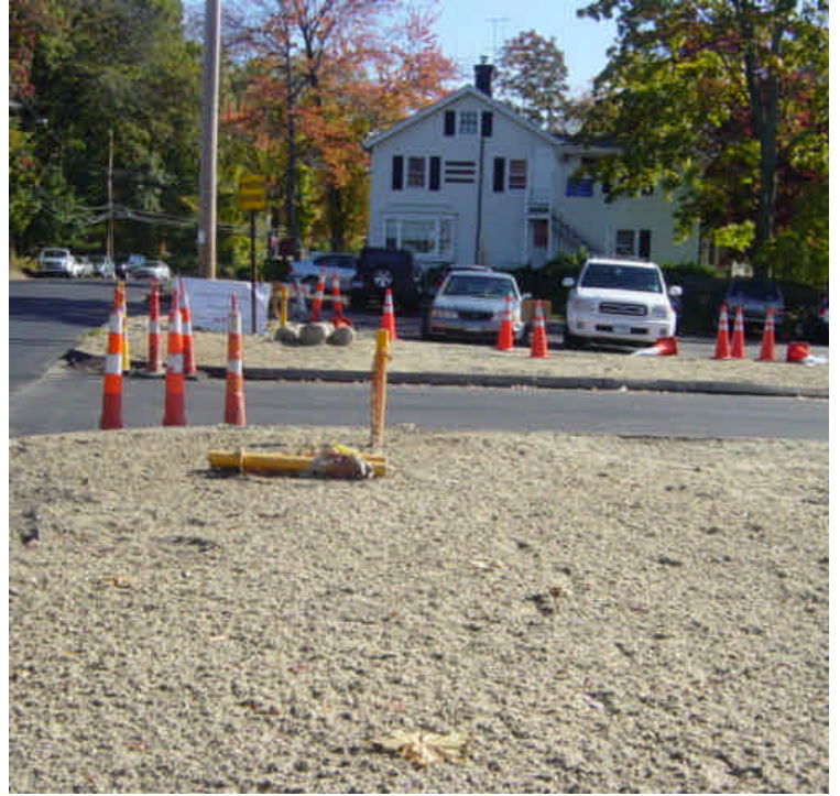
Restoration efforts have been completed near vault #28. The area remains hydroseeded. Monitor for grass cover.
