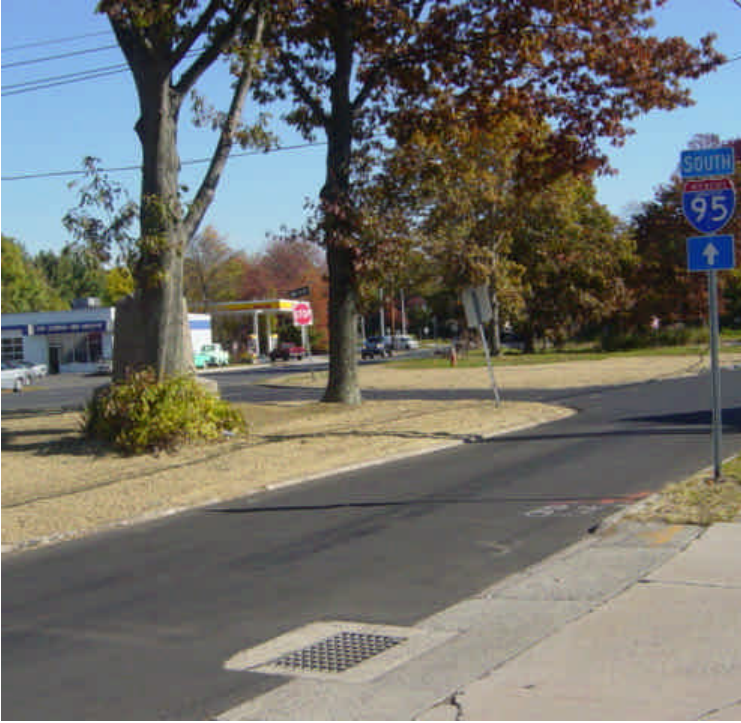
The area near sta. #463 remains restored and hydroseeded. Monitor for grass cover.
