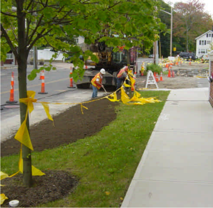
Restoration efforts were observed near sta. #469-470.
