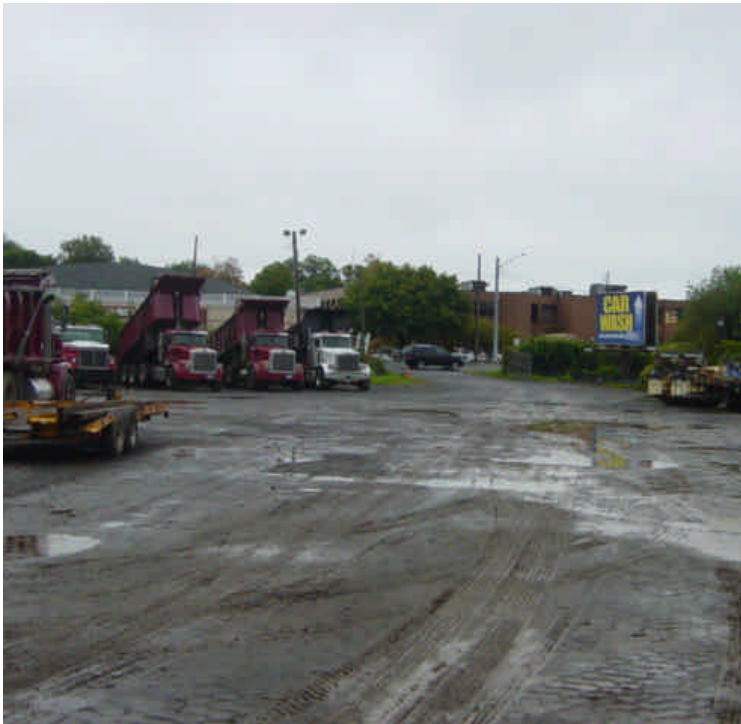
The Kings Highway yard remains in use, but materials and equipment are beginning to demobilize. Portions of the perimeter fence are deteriorating and need maintenance.
