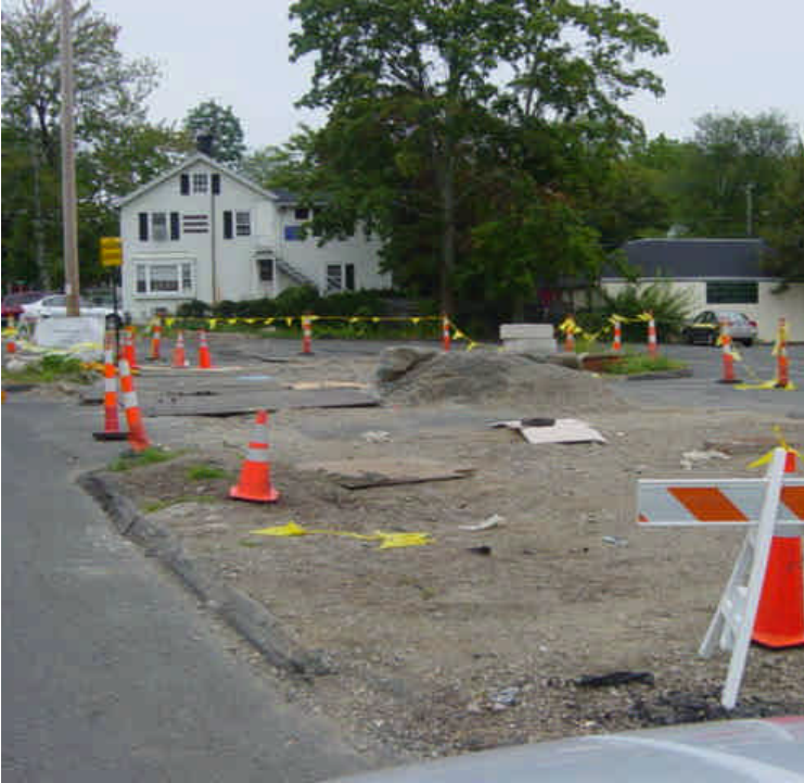
Tie-in work continues near vault #28.
