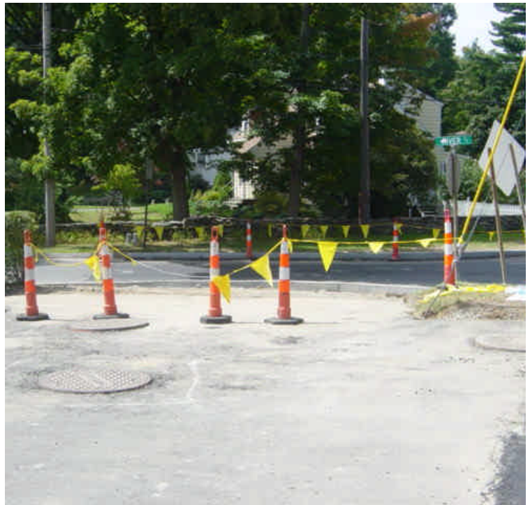
Curbing had been restored near sta. #504-505. near vault #30.
