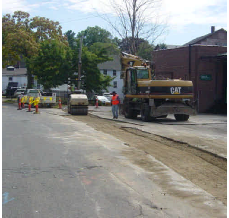
Backfilling and paving operations were underway near sta. #480-482.
