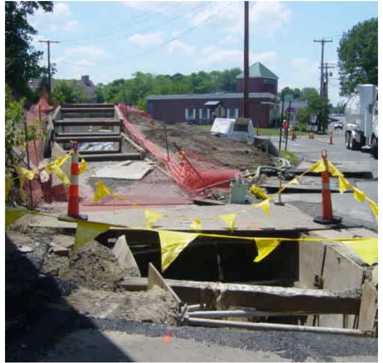
Trenching continues near sta. #462-465. Steel plates covered parts of the trench. Dewatering was ongoing at the time of the inspection.
