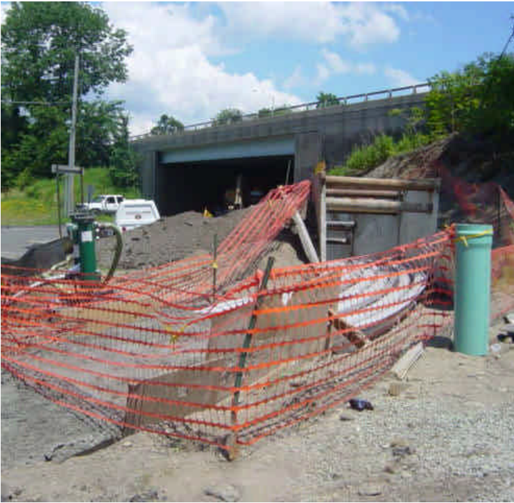
Trenching continues near sta. #462-465. Steel plates covered parts of the trench. Dewatering was ongoing at the time of the inspection.
