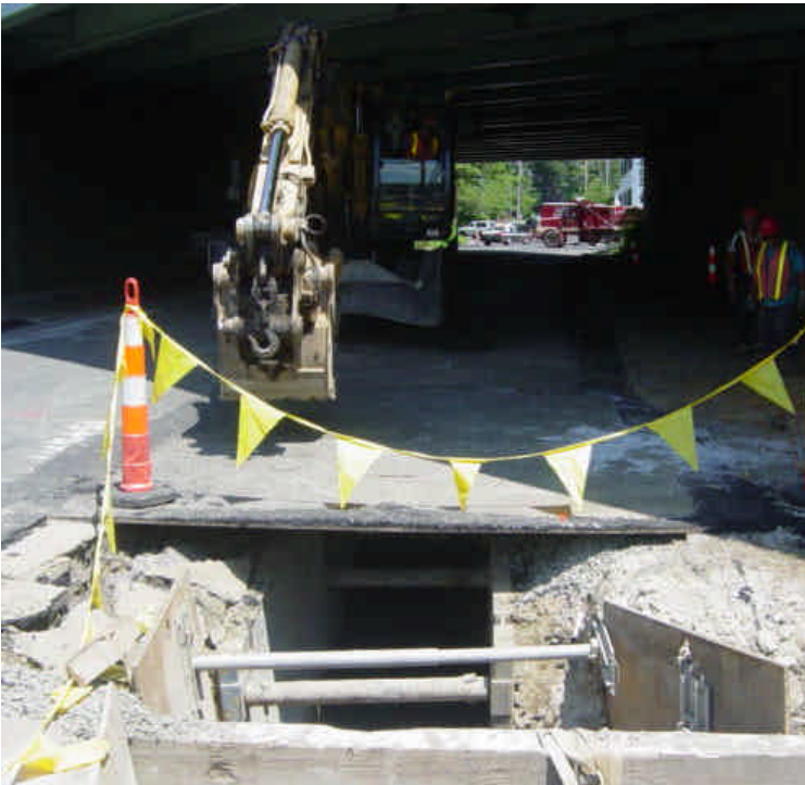
Trenching continues near sta. #466.
