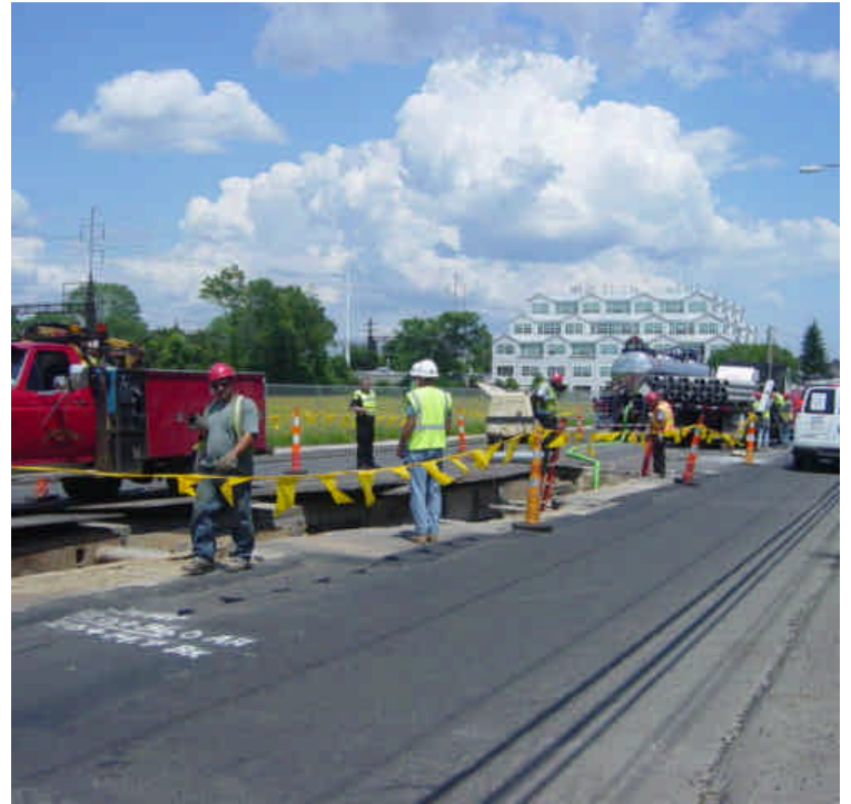
Conduit repair work was ongoing at sta. #519-520.
