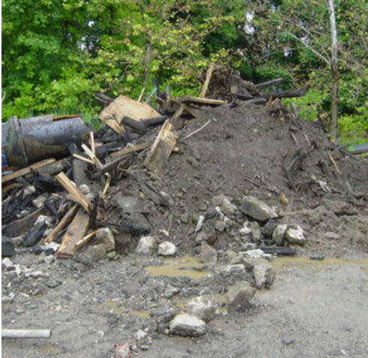
In the King's Highway lay-down yard soil and additional debris material has been mixed with the railroad tie debris which had been previously sorted for disposal. Conduit and other materials have been piled or spilled on the perimeter silt fence which needs repair in several areas.
