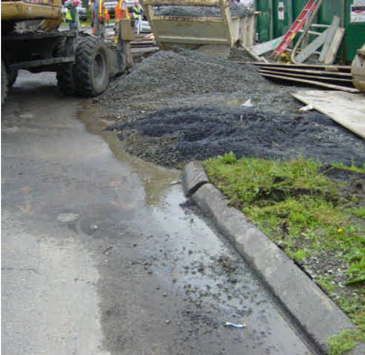
Crews were trenching near sta. #462-464 to realign the conduit. Deawtering activities were ongoing. The site was very muddy but generally well contained. A minor amount of sediment was being tracked onto Old Post Road (Rte 1) from vehicles as they exited the median area. A small amount of turbid runoff was flowing along the curbline and into the downstream catch basin.
