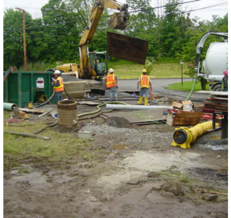
Crews were trenching near sta. #462-464 to realign the conduit. Deawtering activities were ongoing. The site was very muddy but generally well contained. A minor amount of sediment was being tracked onto Old Post Road (Rte 1) from vehicles as they exited the median area. A small amount of turbid runoff was flowing along the curbline and into the downstream catch basin.
