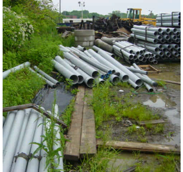
In the King's Highway lay-down yard soil and additional debris material has been mixed with the railroad tie debris which had been previously sorted for disposal. Conduit and other materials have been piled or spilled on the perimeter silt fence which needs repair in several areas.
