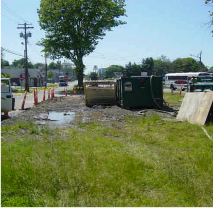
Crews were dewatering near sta. #462-464 in preparation for trenching work to realign the conduit. During dewatering activities, the filters appear to have clogged and an overflow occurred. A small amount of turbid runoff was flowing along the curbline and into the downstream catch basin.
