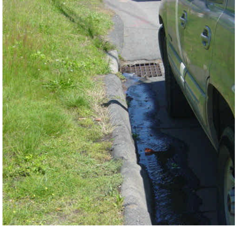
Crews were dewatering near sta. #462-464 in preparation for trenching work to realign the conduit. During dewatering activities, the filters appear to have clogged and an overflow occurred. A small amount of turbid runoff was flowing along the curbline and into the downstream catch basin.
