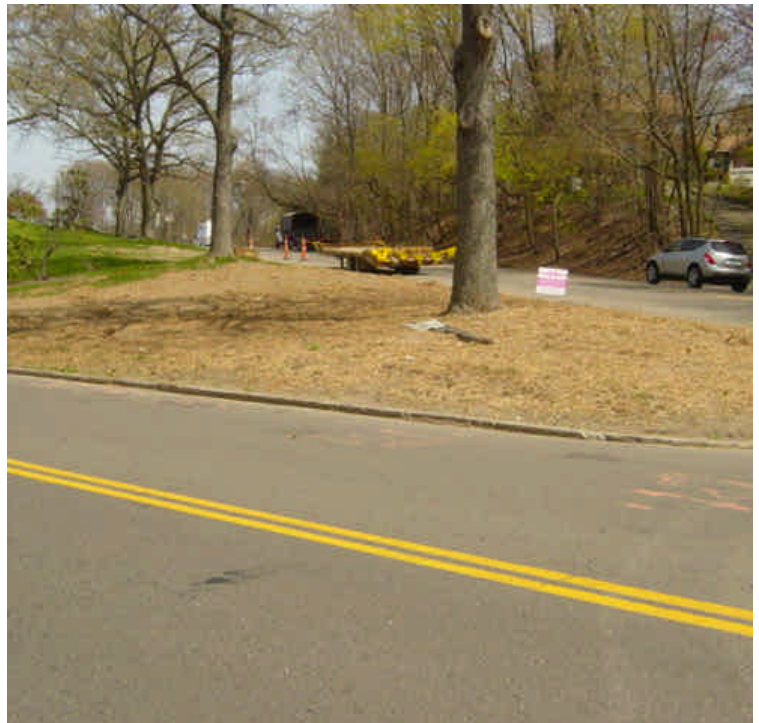
Seed and mulch have been applied over the previously exposed soil on the median near sta. #495.
