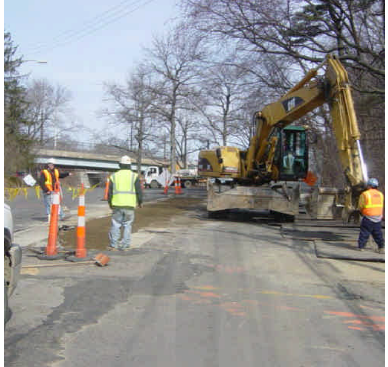
Both photos (above) show trenching and backfilling activities continuing near sta. #488-493.
