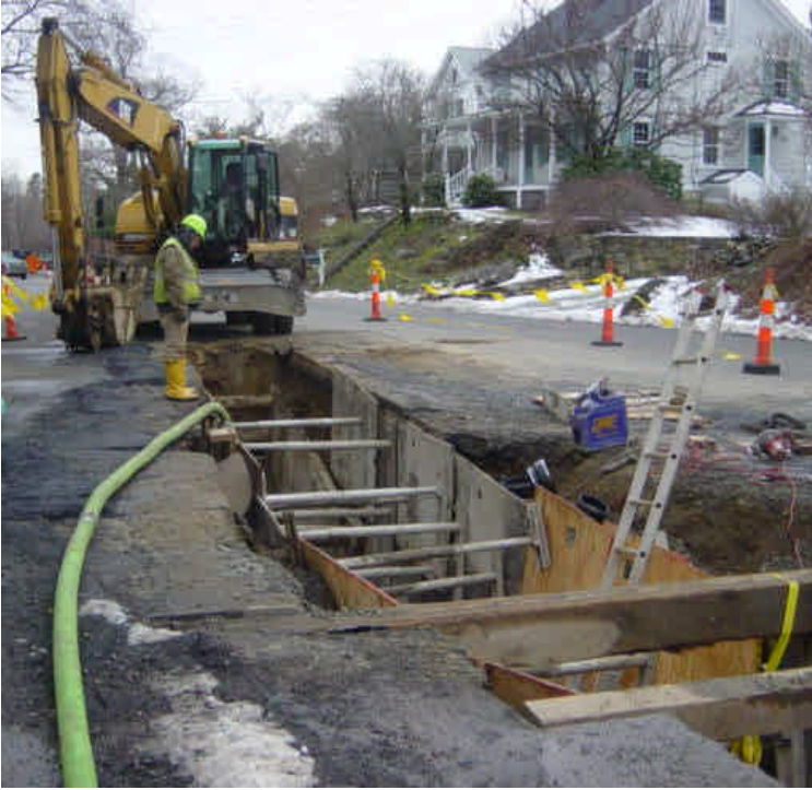
At sta. 491-493 on Pequot Avenue, dewatering and trenching were in progress.
