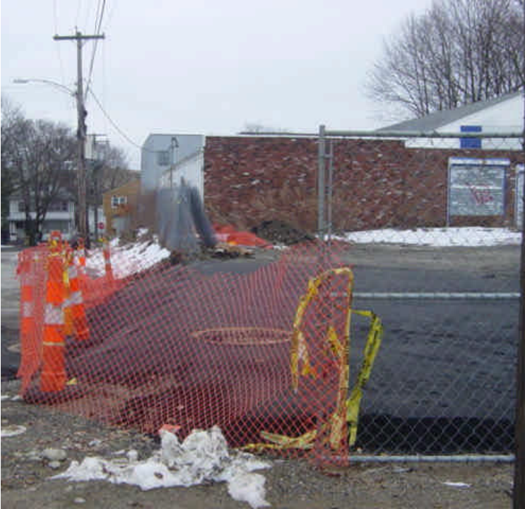
Vault #42 has been paved near Fairfield Avenue in Bridgeport.
