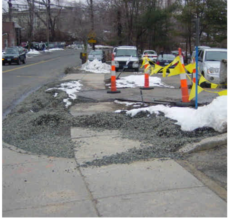
Near the corner of Pequot Avenue and Old Post Road, stone has been installed to stabilize previously exposed soil near the bank parking lot.
