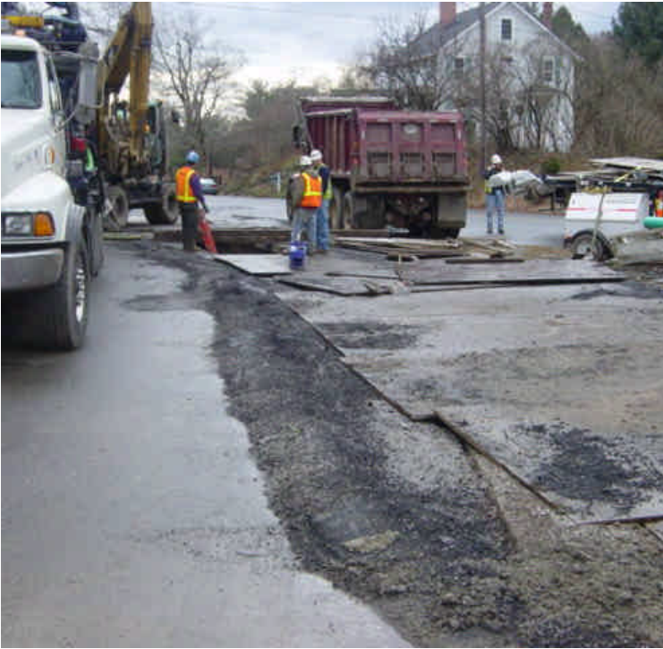
Trenching activities continue along Pequot Ave. near sta. #493 to 494. A temporary bituminous berm was created along the edge of the steel road plates to divert runoff away from the trench. Excavated material from the trench was being placed into a dump truck. Ground water from the soil was draining out of the back of the truck. The turbid runoff was flowing along the curb line for approximately 250 feet before reaching a protected catch basin. During the inspection, a contractor Supervisor was called out to the site to address the multiple issues in this area.
