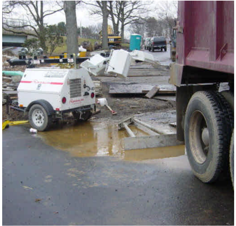
Trenching activities continue along Pequot Ave. near sta. #493 to 494. A temporary bituminous berm was created along the edge of the steel road plates to divert runoff away from the trench. Excavated material from the trench was being placed into a dump truck. Ground water from the soil was draining out of the back of the truck. The turbid runoff was flowing along the curb line for approximately 250 feet before reaching a protected catch basin. During the inspection, a contractor Supervisor was called out to the site to address the multiple issues in this area.
