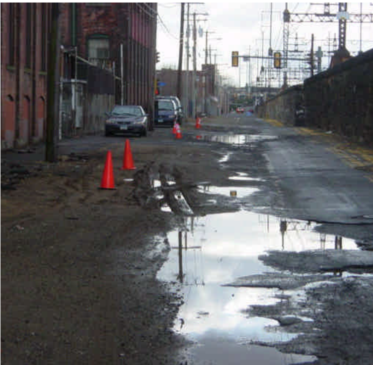
Some ruts were noted along the shoulder of Railroad Ave. near sta. #737. Ruts were likely from normal traffic but more hard pack or gravel may be needed here.
