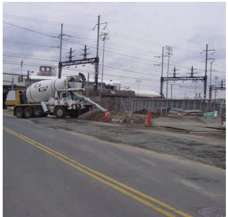
Concrete washouts were being performed properly in a contained area.
