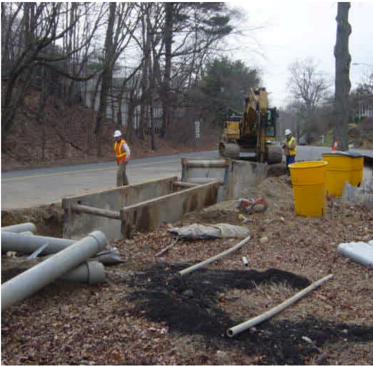
Trenching activities continue along Pequot Avenue near sta #494-495.
