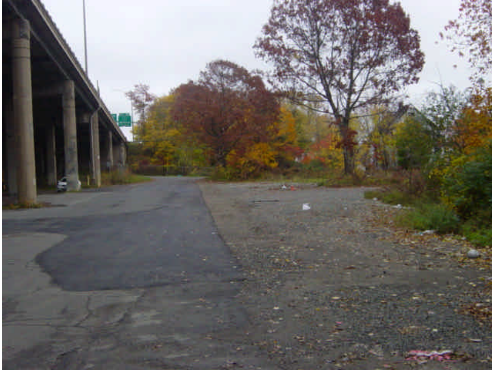
Work in the area of sta #1015-1020 is complete and the area was paved.
