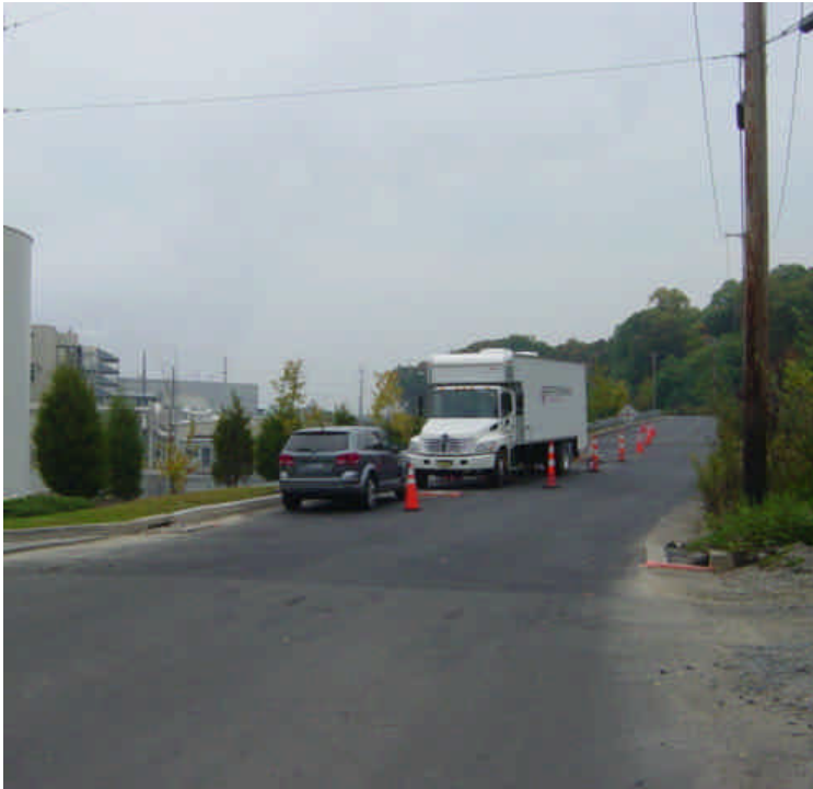
Electrical contractor was on site at vault #6.
